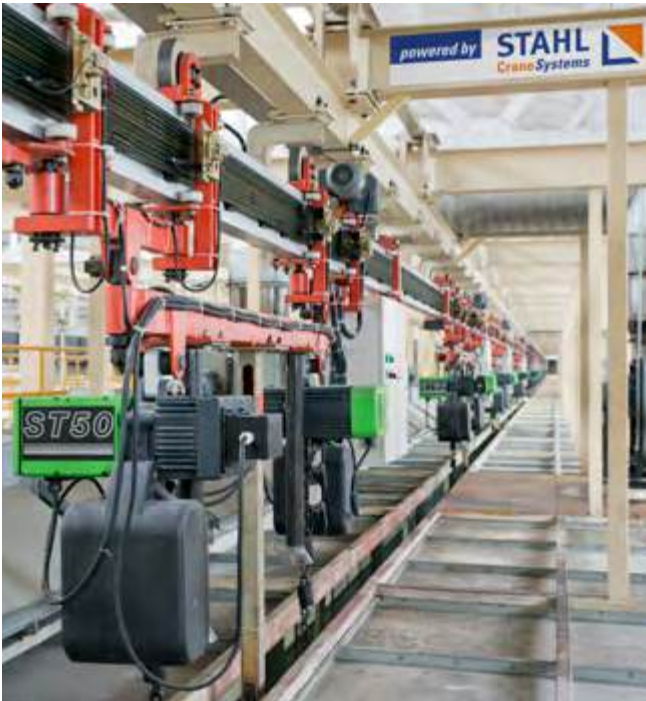
Two ST 50 chain hoists acting in tandem lift complete car bodies and transport them along the assembly line.
