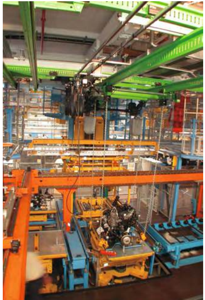
Synchronous lifting for four-point load attachment by coupling the chain hoists.
