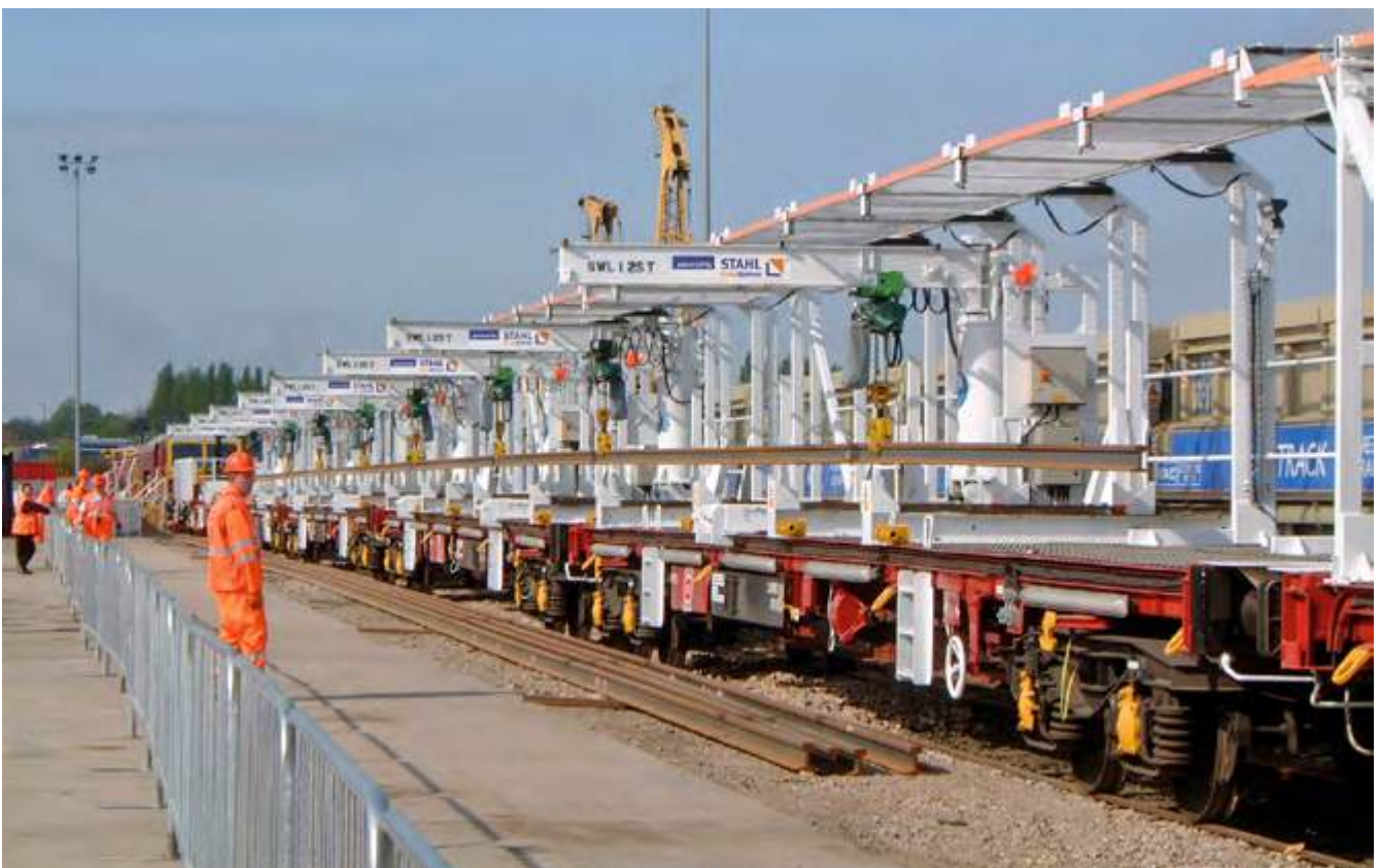
A number of ST chain hoists are used in the maintenance and replacement of train rails in England. All the hoists are equipped with customised load lifting equipment. They are centrally controlled to ensure that they work in synch. They are disconnected by a gear limit switch, reliably limiting the lifting process.
